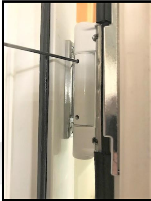
Figure 17: Removing Cover Plates
