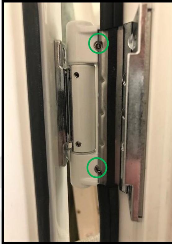
Figure 25: Adjusting Compression Set Screws
