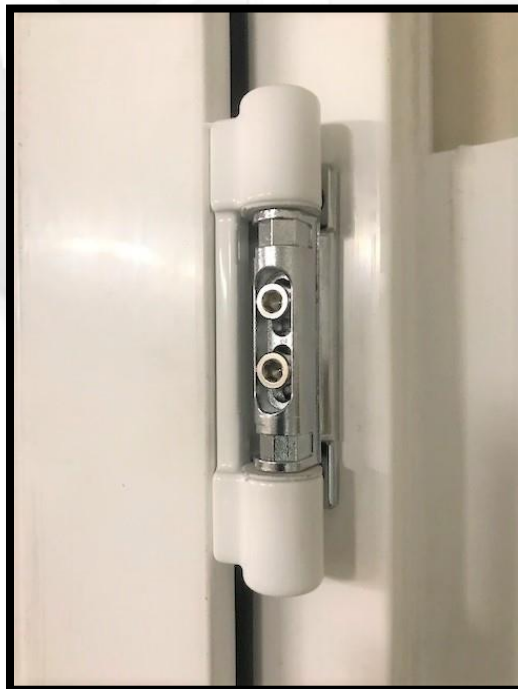
Figure 18: Exposed Socket Head Cap Screws
