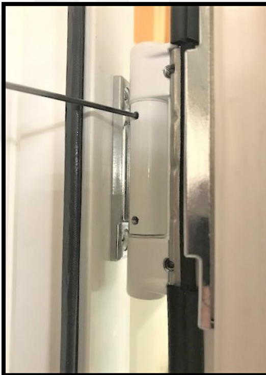
Figure 24: Tightening Cover Plate Screws Set Screws
