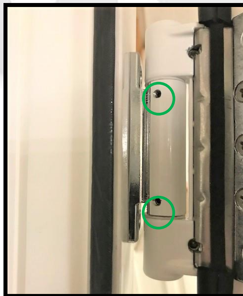
Figure 16: Cover Plate Set Screws
